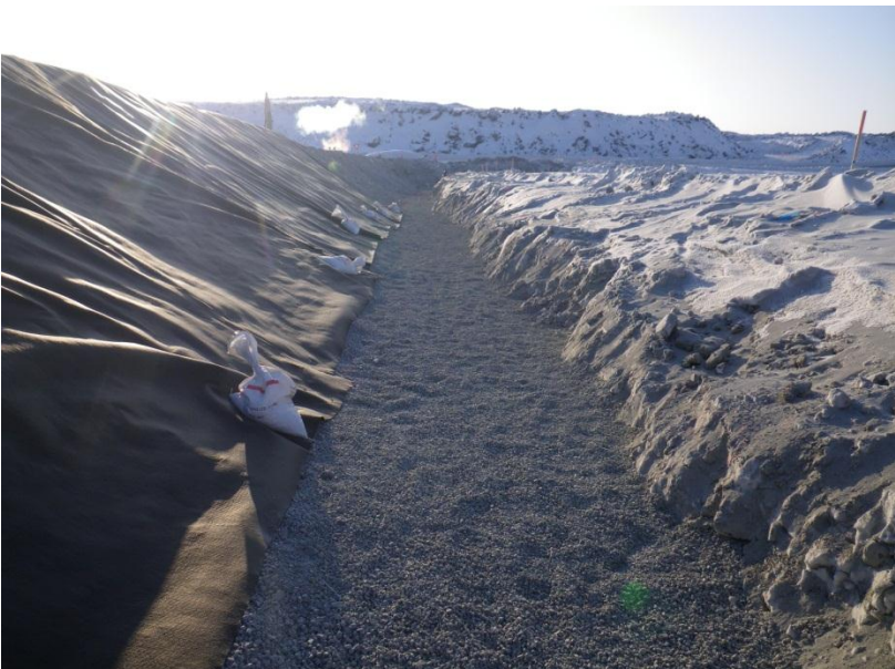
Photo 8: Bentonite placed in base of key trench and under HDPE geotextile.
