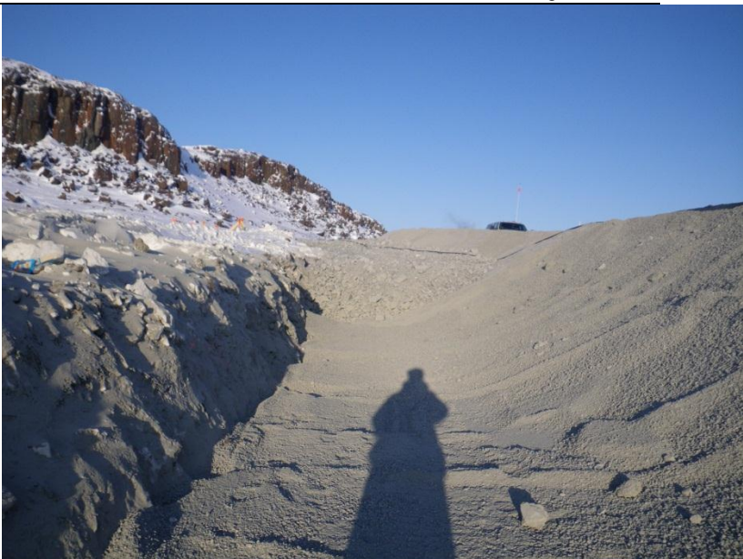
Photo 9: Over liner crush placed from 160 to 100, looking east along berm. Face of ROQ front visible.
