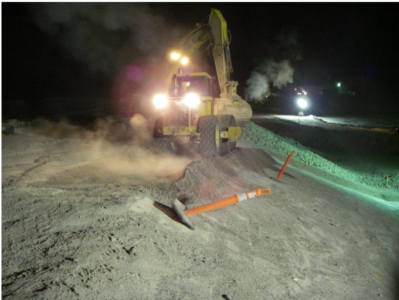
Photo 13: Placing and compacting the last of the FCM at approximately station 0+70.
