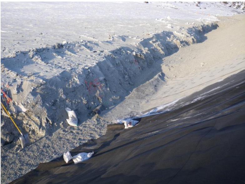
Photo 10: Wrinkle in HDPE liner at approximately station 100.
