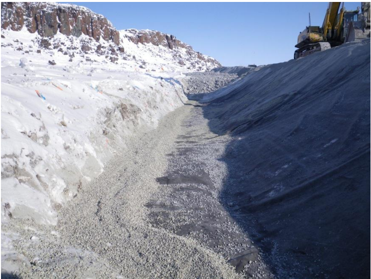
Photo 11: Bentonite 'plug' placed from 100 to 160, photo looking east.
