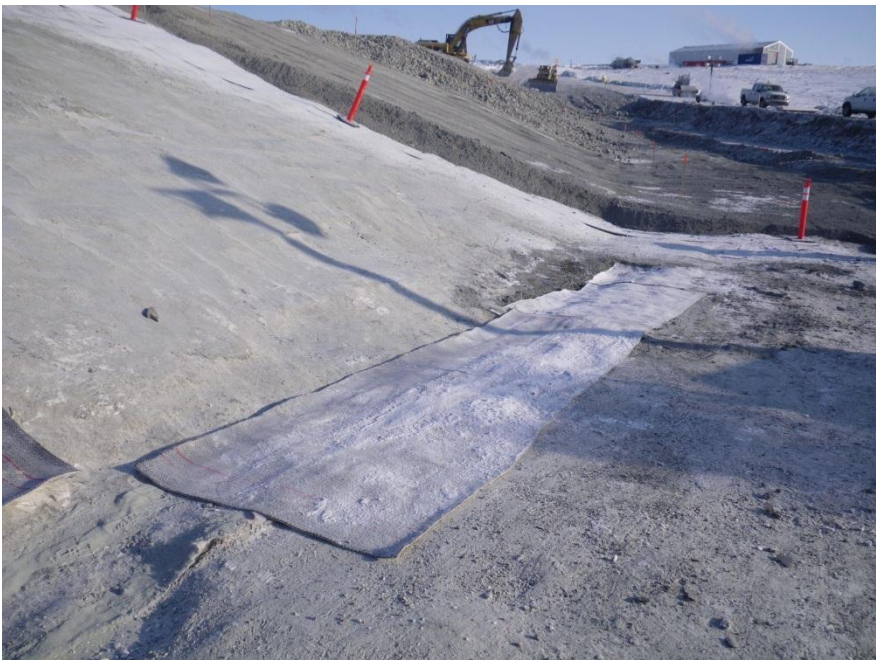
Photo 4: large patches placed over the GCL liner near station 0+75.
