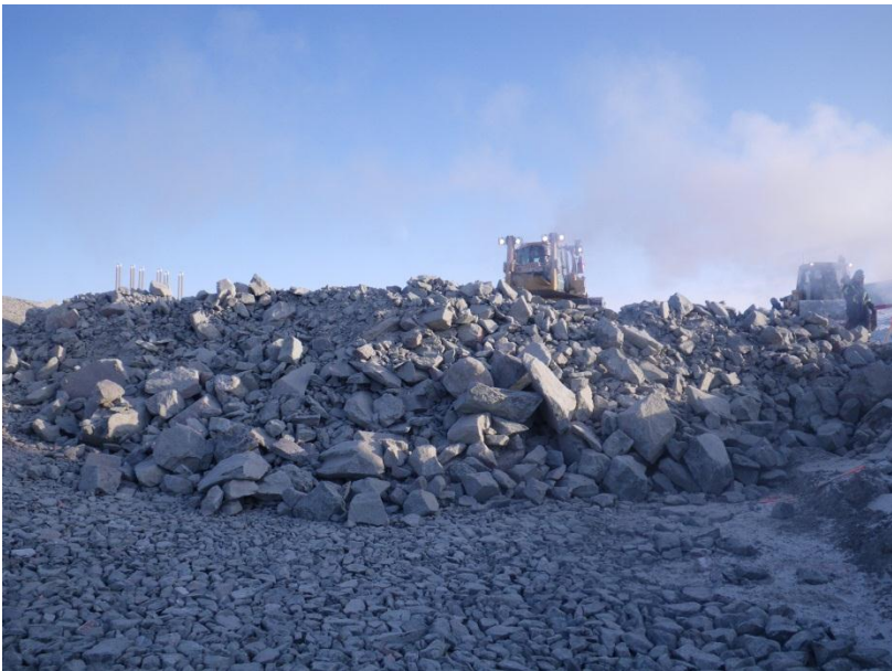
Photo 12: ROQ placement at the north dam.
