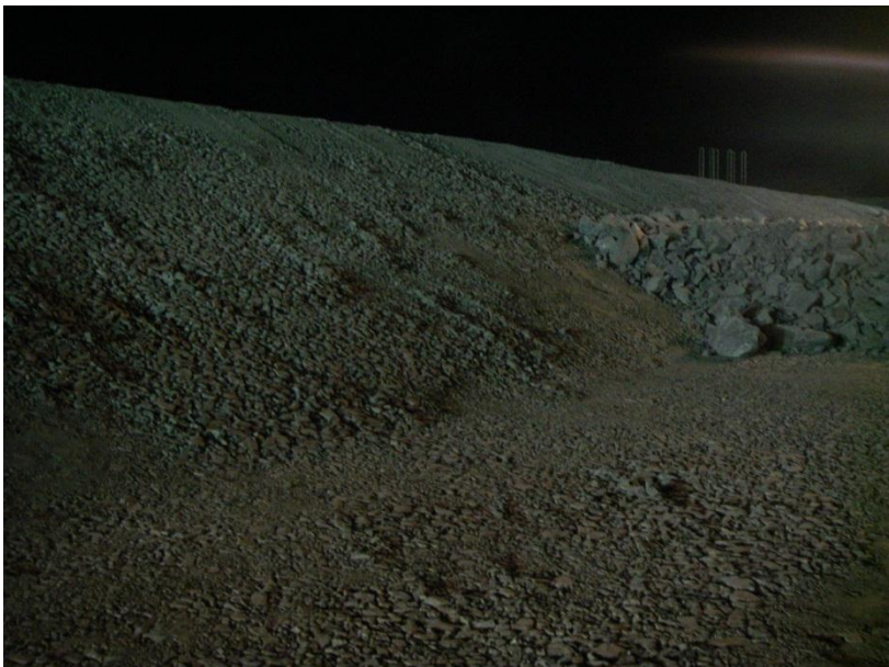
Photo 15: Compacted .Transition material on the upstream slope. Photo looking north-west from Sta. 1+00. Note the lift of ROQ in the background.
