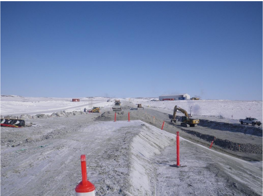
Photo 5: Photo looing north east at the transition and ROQ placement on the North Dam.
