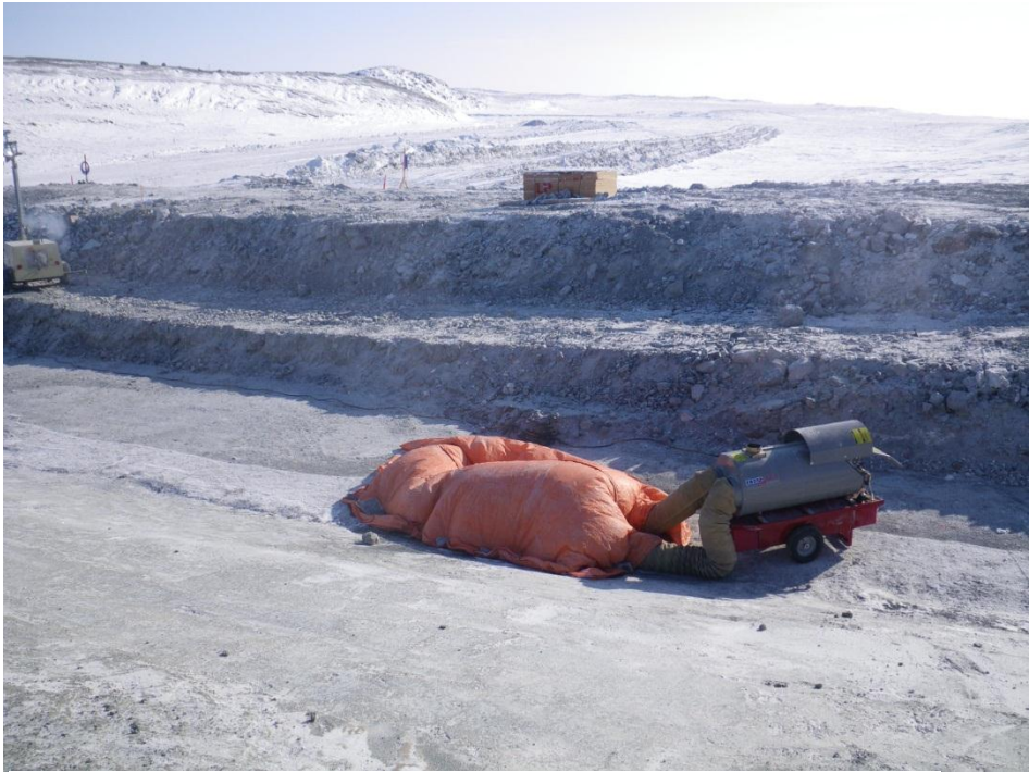
Photo 6: Heating and hoarding on the lower GCL.
